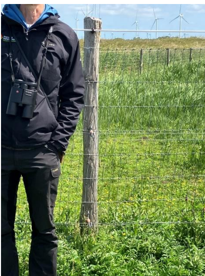
Figure 3: Example, Permanent fence, Mesh UK imported, 5x15 cm, 120 high + 50 cm parallel to ground, additional 3 wires conductive, top wire with improved visibility. Posts has spikes/pins,
